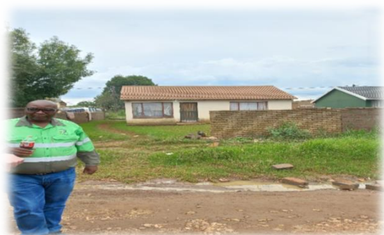
Picture 7: Disaster Management officials conducting damaged assessment
